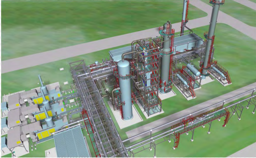
3-D model of a gas fractionating plant
