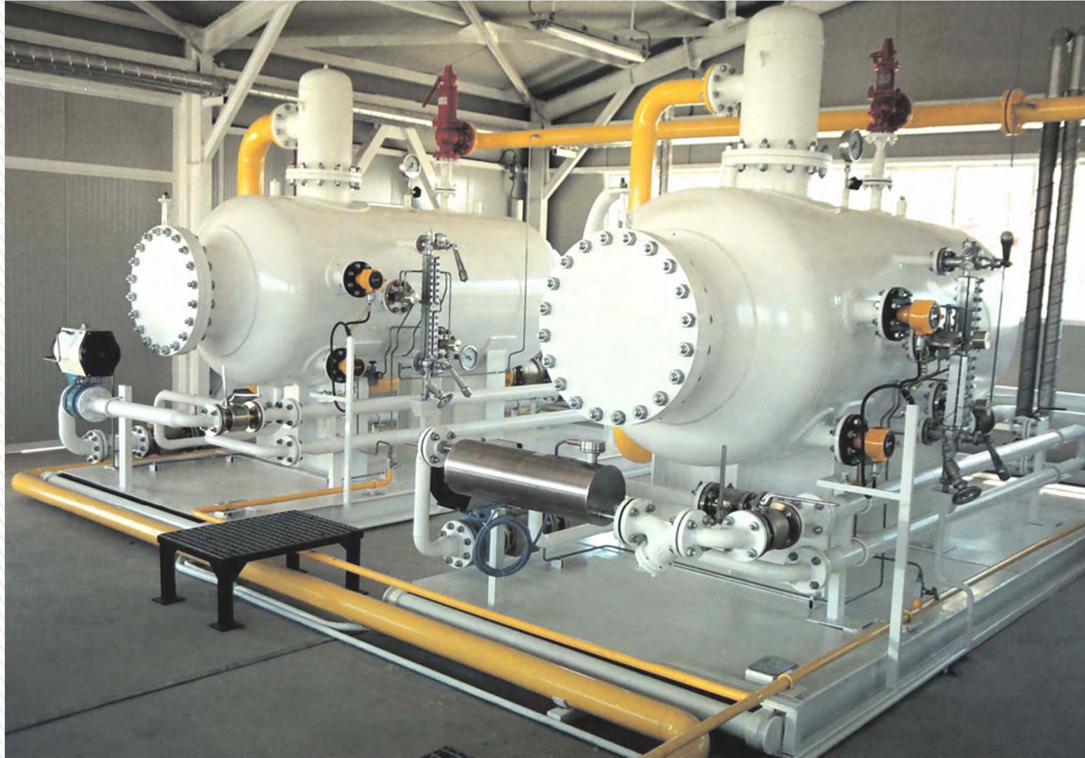
Bi-phase calibration separators
